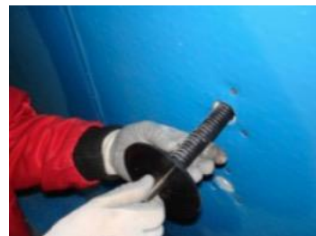
Figure 10. Ancrage PEHD
